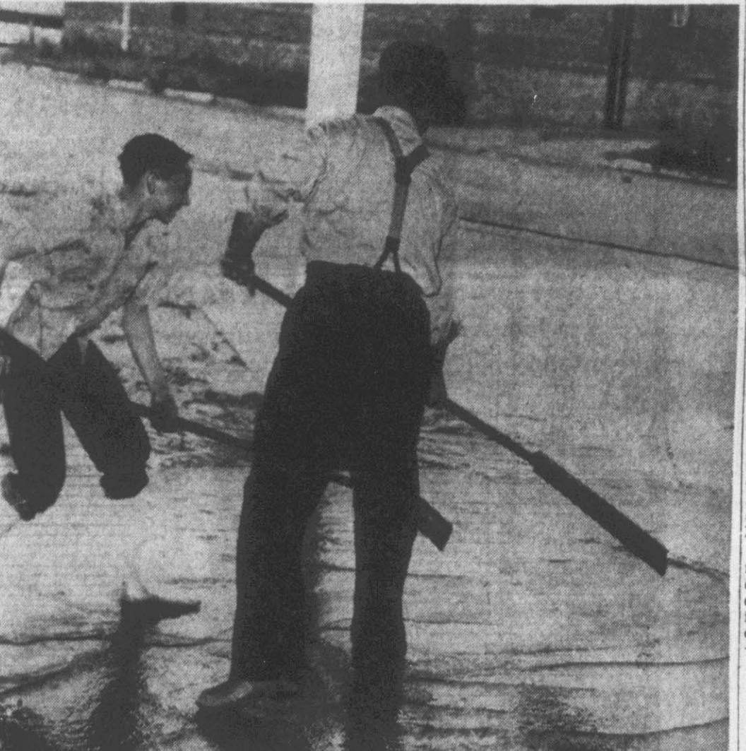
Traffic Blocked; Fire Sub-Station Is Engulfed Rain Floods City Streets
