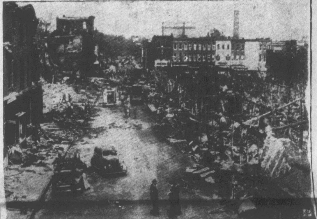
BLOCKBUSTER? NO, FIRE!—This is all that remained of the blocklong Lafayette Market (right) after an early morning 12-alarm fire burned out 12 other buildings and damaged 30 in Baltimore. A shifting wind sent a sheet of flames across the street where 15 three-story row houses were completely burned out. At the height of the fire, eight of the 15 houses (shown at left) collapsed in a shower of bricks. There was no immediate estimate of the damage, or the cause of the blaze. (AP Wirephoto)
