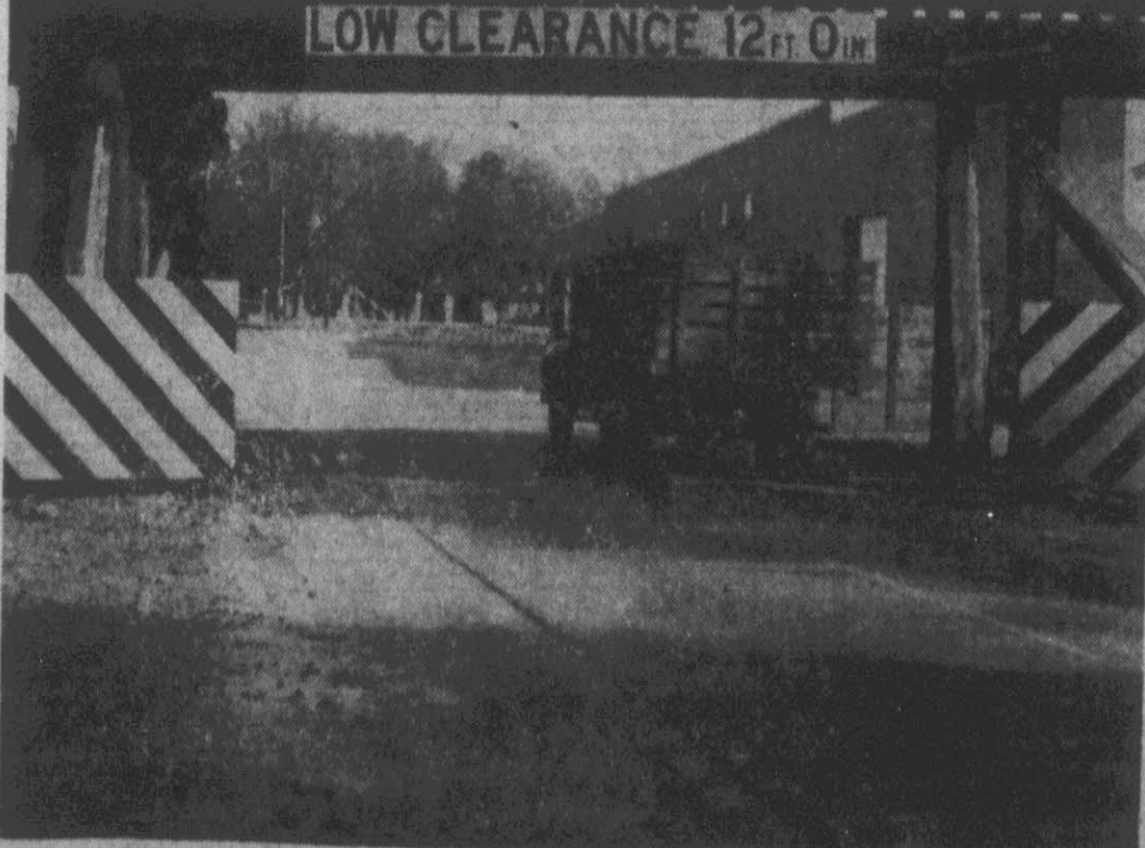
TRUCK GAP HEIGHTENED - The underpass on the New Bern highway which has been a "trap" for large trucks in recent years is now in the process of being heightened by the State Highway Commission and the Norfolk and Southern Railroad. When completed, the underpass will no longer endanger unloaded, large vehicles. (Reflector Photo by Roy Hardee)
