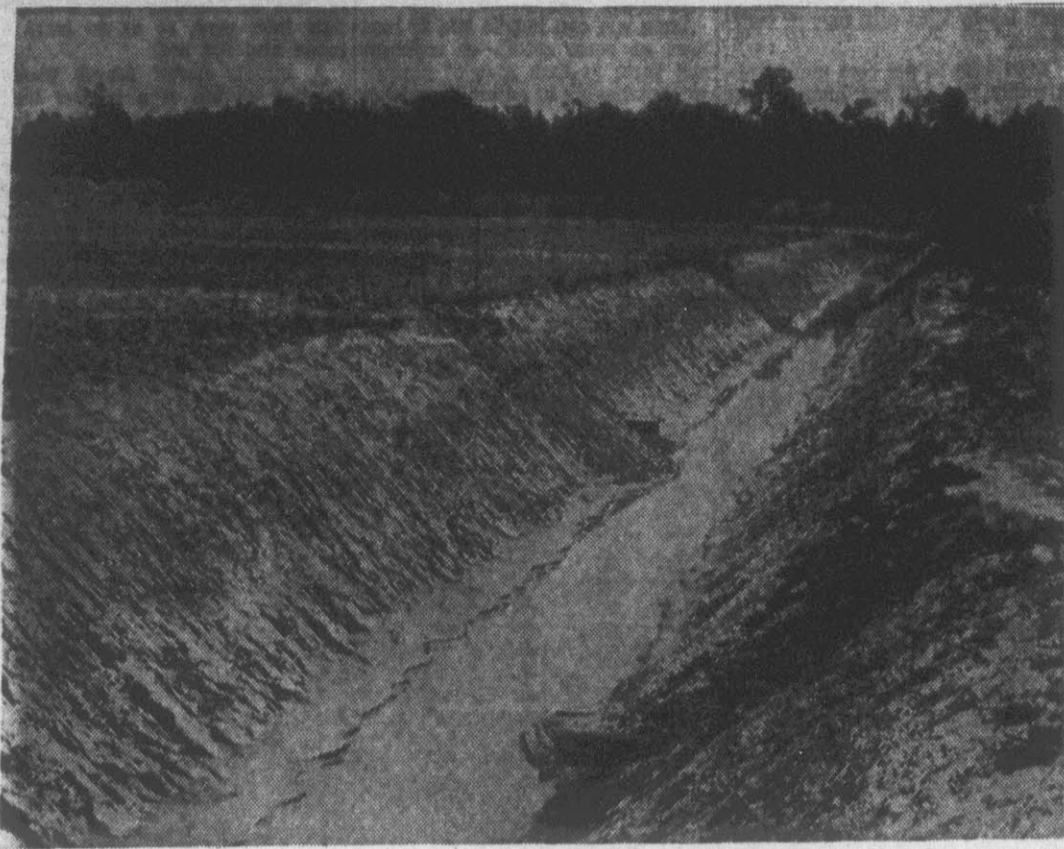
SOIL CONSERVATION GAINS —The Soil Conservation program swept ahead last year as construction of open drainage ditches, installing of drain tile, such as shown above increased. By the use of such ditches which carry off the excess water, other wise unusable farm land is reclaimed and made to pay off in increased crop production. (Reflector Photo by Roy Hardee)
