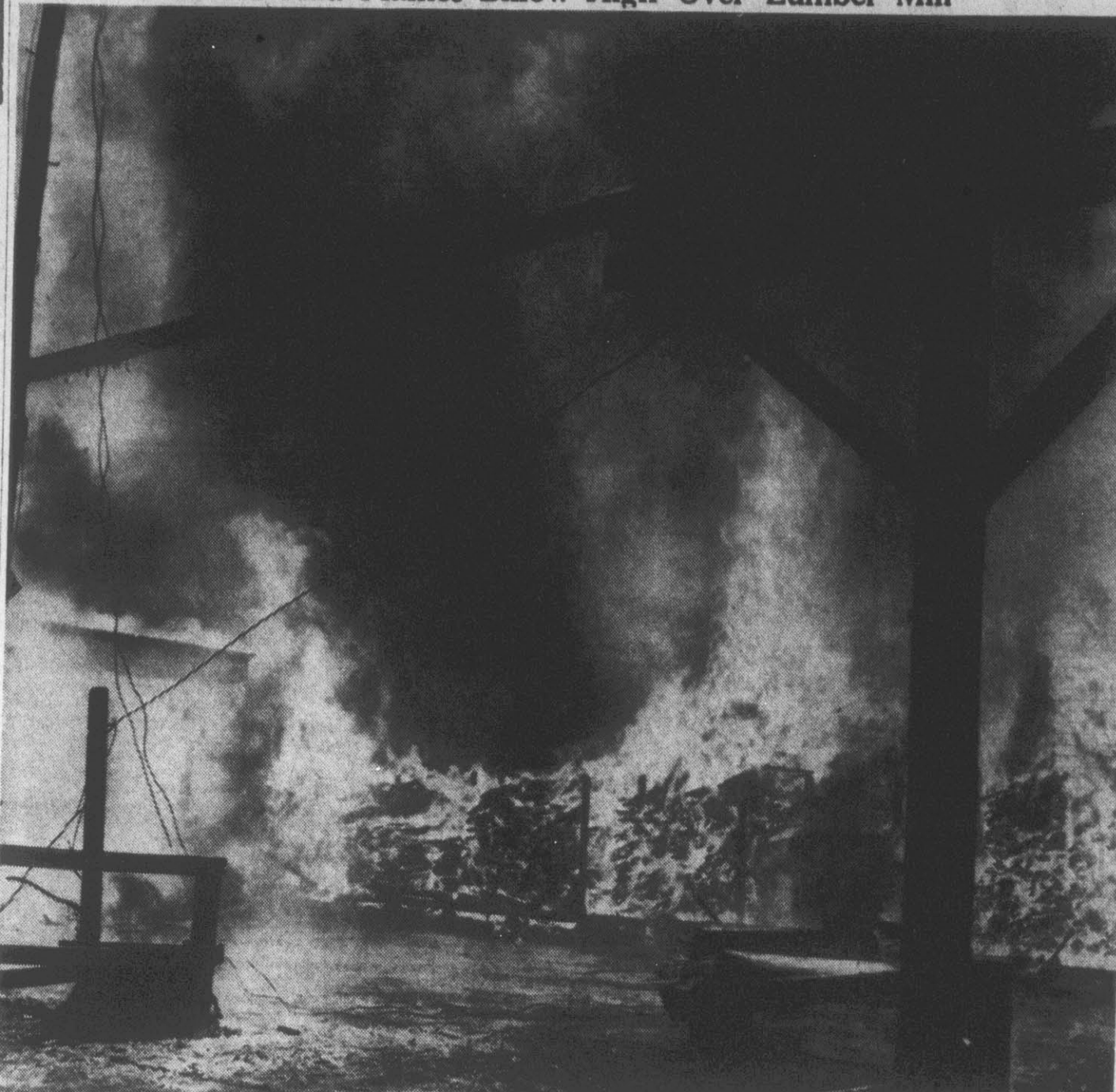
Leaping flames and billowing smoke are shown pouring from the devastating blaze which swept through North Side Lumber Company here late this morning. Flames swept through the planing mill and later caused the walls of the dry kiln (pictured at left) to collapse. It was estimated that more than 300,000 feet of lumber were destroyed in the blaze. (Reflector Photo by Roy Hardee)
