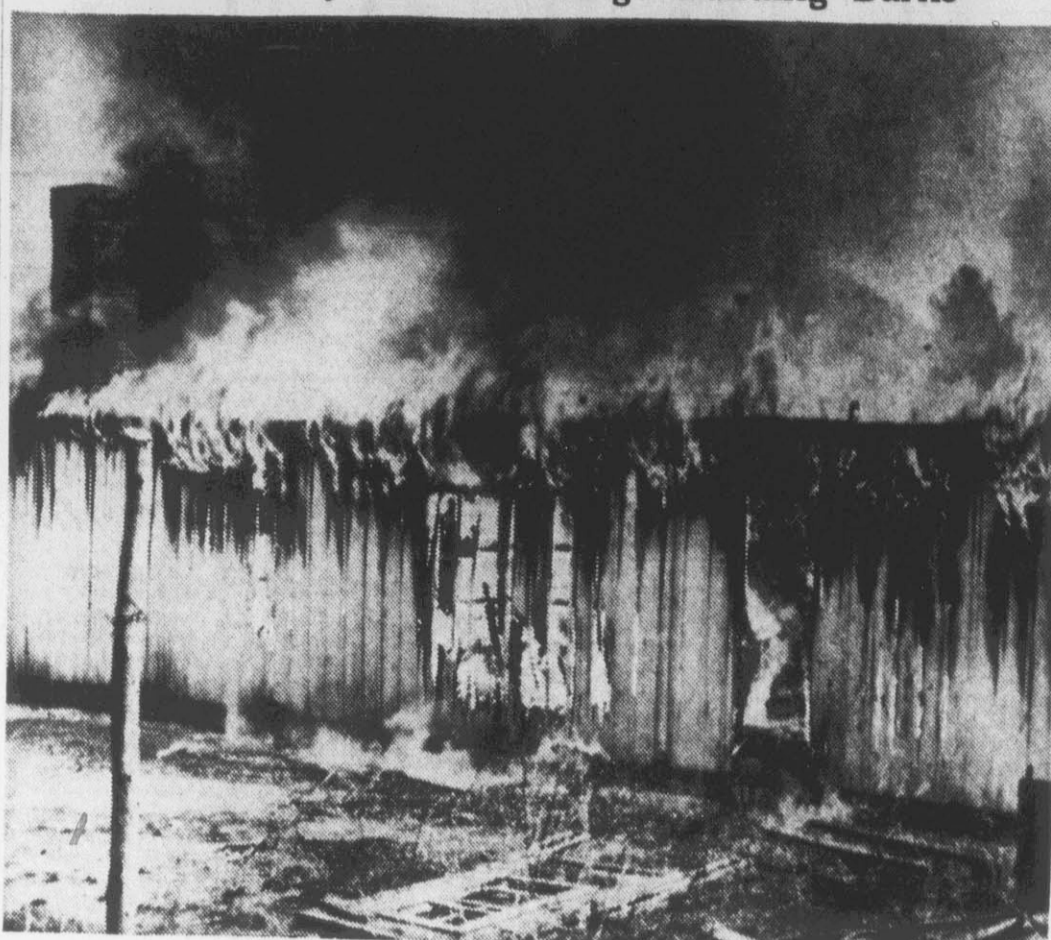
Flames quickly engulfed a storage building at Brookgreen school early this afternoon. It was discovered by Principle James A. Vinny and a group of students working in the school garden near the building. A reported $6,000 insurance was said to cover the building and contents. (Reflector Photo by Roy Hardee)
