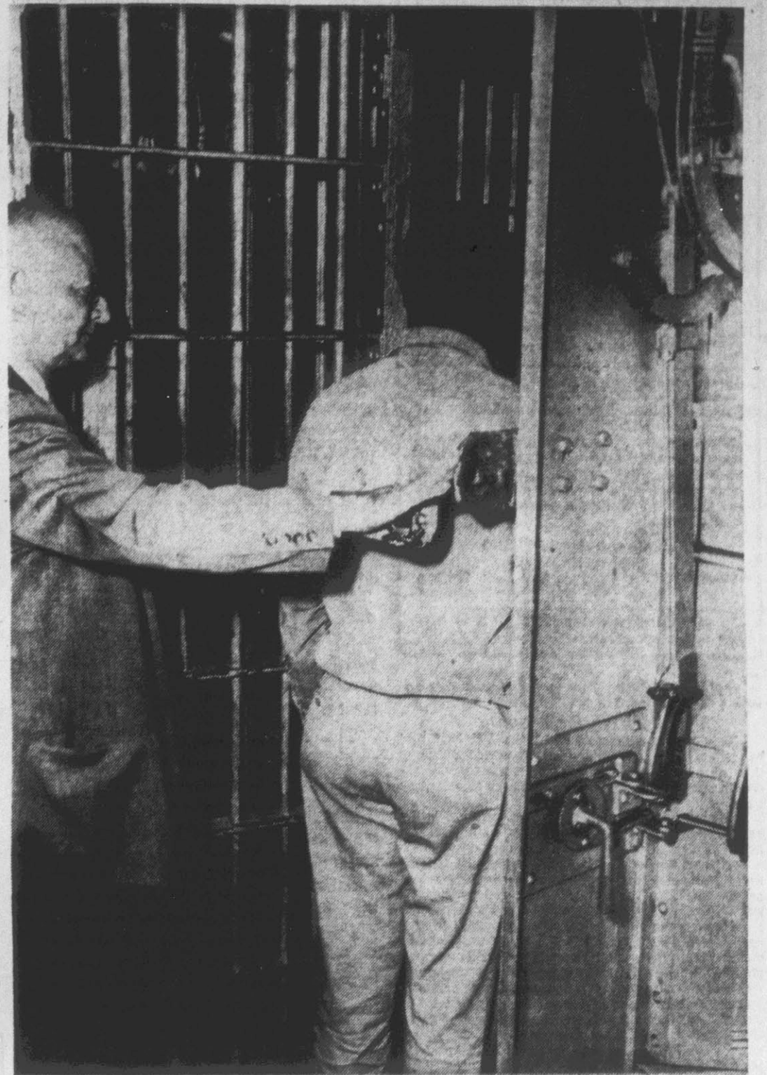
More than 7,500 persons have been placed under lock and key by jailer Leggett since he assumed duties as the first full-time jailer 16 years ago. Here, Leggett opens the door of a cell block to admit a prisoner.
