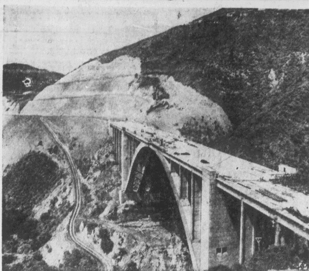
GOING ROUND THE MOUNTAIN —Work nears completion on pre-stressed concrete bridge between La Guaira and Caracas, Venezuela, in foothills of Andes. Bridge is 1,930 feet long, has 500-foot span 220 feet above creek and is one of longest of its type in world.
