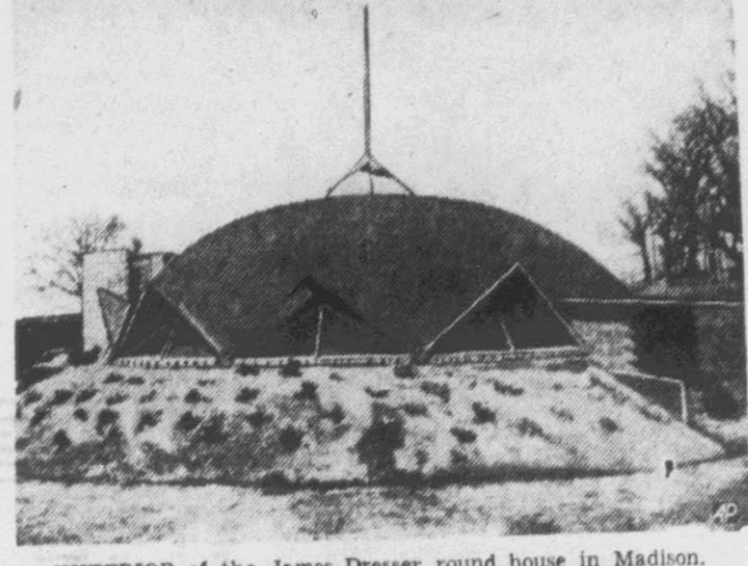
EXTERIOR of the James Dresser round house in Madison.
