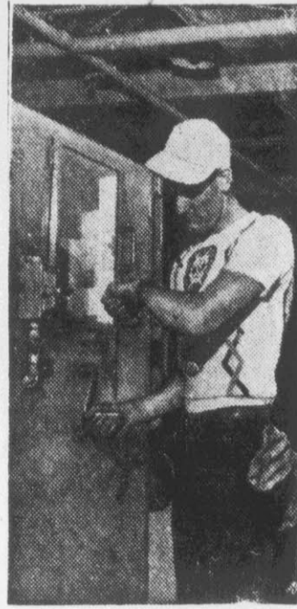
INDUSTRY —An atomic tracer is injected into a pipeline. It is used to trace the progress of liquids being pumped through the line.
