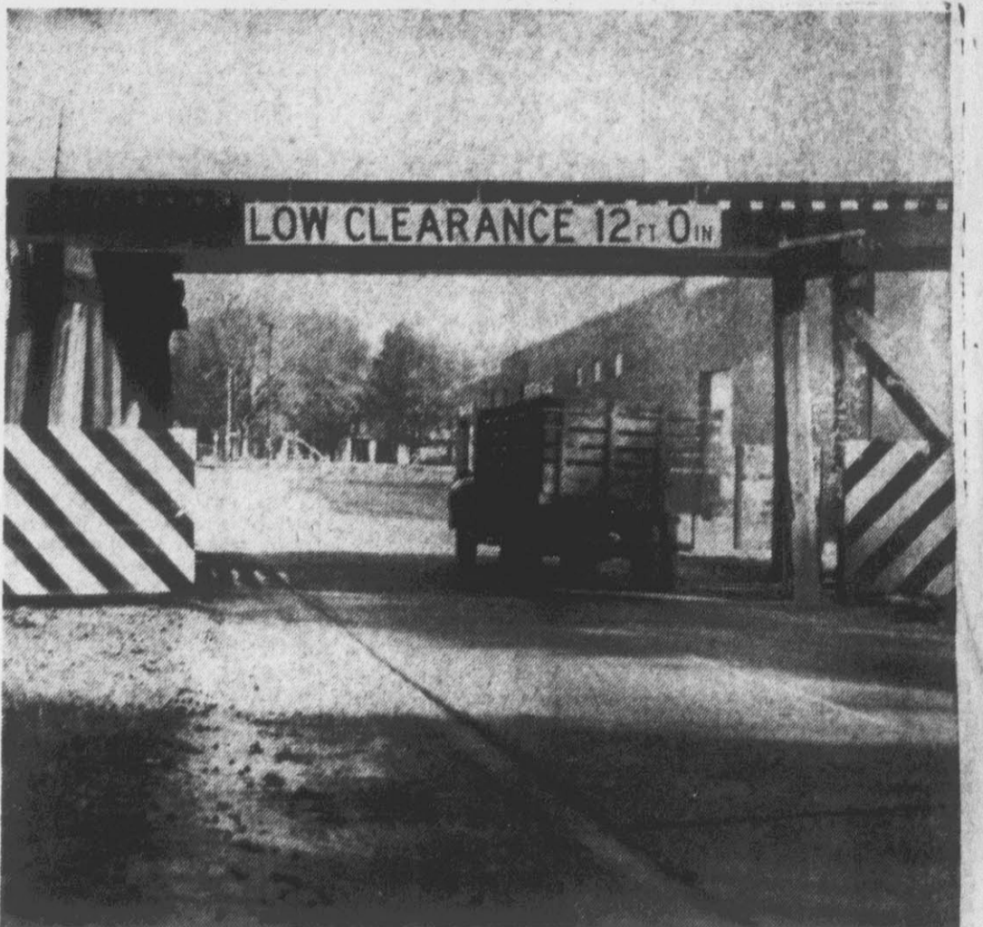
The raising of the railroad trestle on Highway 43 was announced this morning. Long an item of controversy, approval has been granted for modifications of the underpass construction, with work scheduled to begin the week of March 9. Cost of the improvements will be shared by the State Highway and Public Works Commission and the Norfolk and Southern Railroad. The low underpass has been the scene of five accidents involving trucks and cars since 1950. (Reflector Photo by Roy Hardee)
