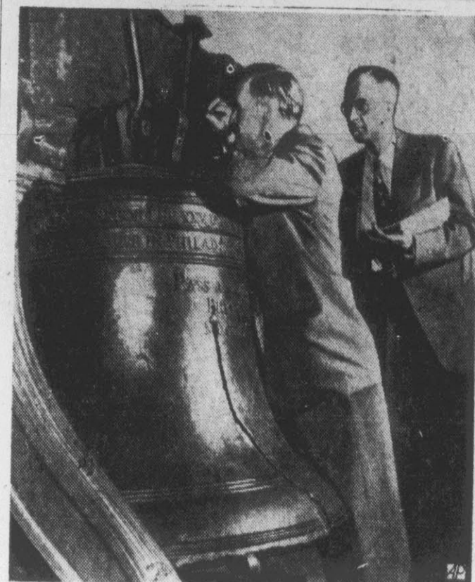
SUPPORT CHECK—Dr. B. Francis Kukachka, left, and Alan D. Freas, wood experts, check the century-old wood beam supporting the Liberty Bell in Philadelphia to determine if the beam can continue to hold up the 2,080-pound bell.
