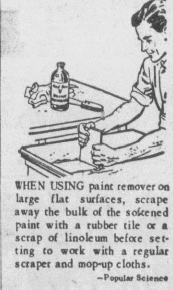
WHEN USING paint remover on large flat surfaces, scrape away the bulk of the softened paint with a rubber tile or a scrap of linoleum before setting to work with a regular scraper and mop-up cloths. —Popular Science
