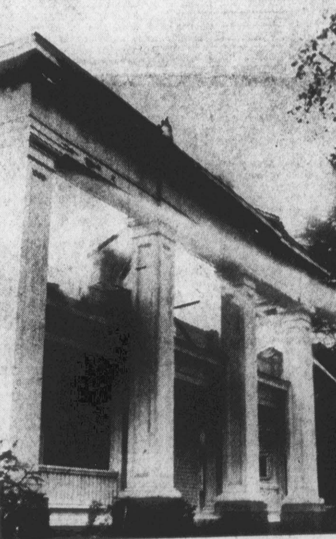
Streams of water were poured between pillars of the grade school's entrance, reaching for the fiery interior. All children were quietly marched to safety well before the flames mushroomed through the entire building. (Reflector Photos by Roy Hardee)
