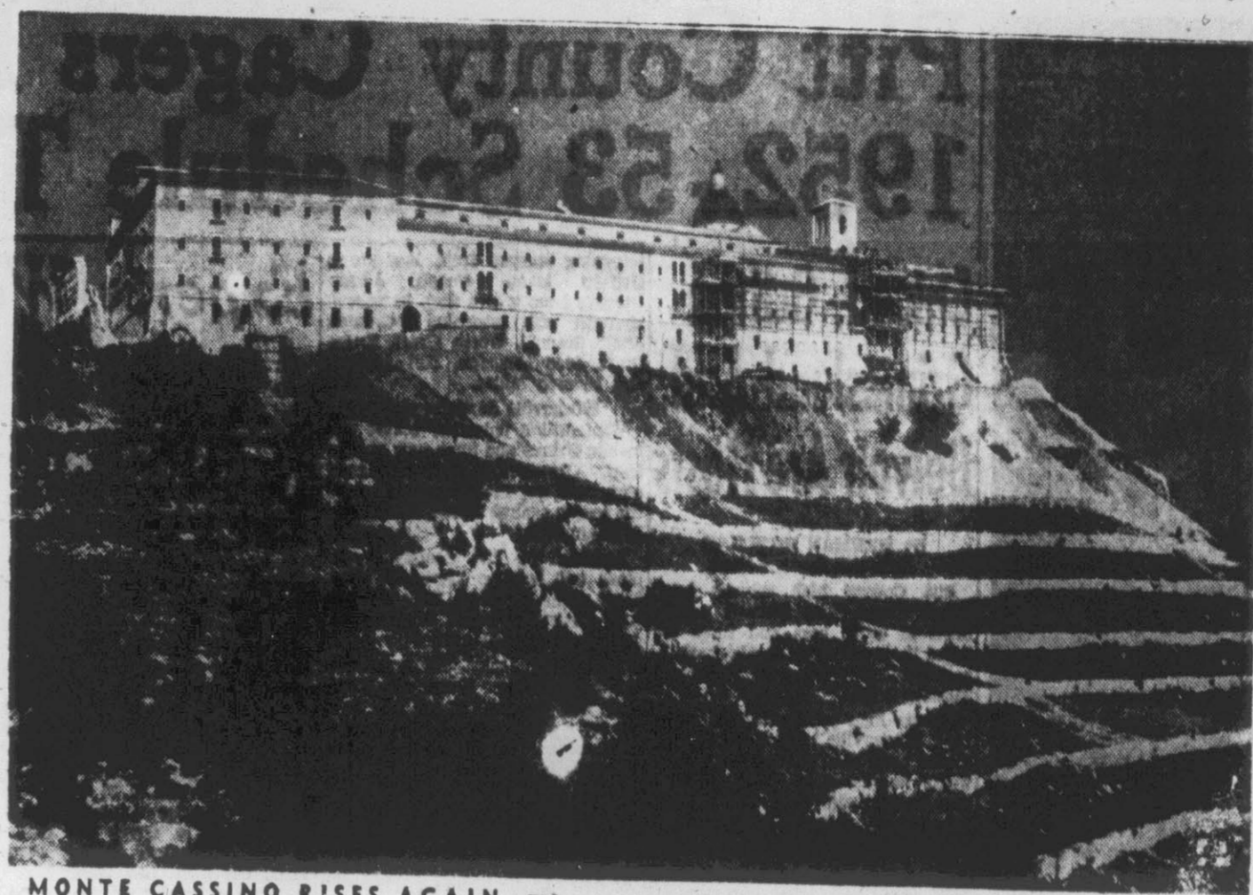
MONTE CASSINO RISES AGAIN—The ancient historic Benedictine Abbey of Monte Cassino, familiar to thousands who fought their way through Italy in World War II, presents this rebuilt face following extensive post-war repairs.
