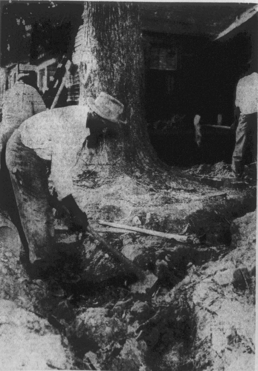
Tree-cutting and other unusual activities are part of the Street Department's everyday chores. Here a tree-trunk is being removed to clear a right of way for the street-makers.
