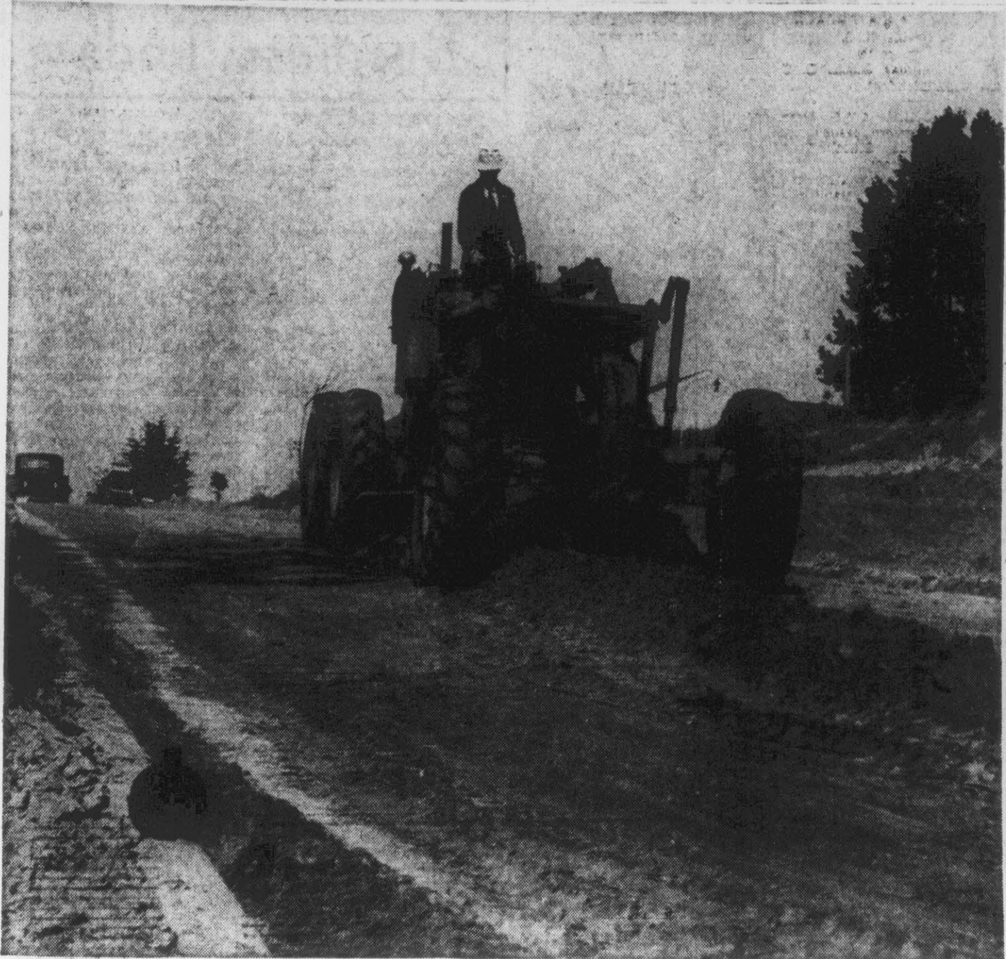
The Street Department's grading machine doesn't have many "days off," and is kept pretty much in use. The big blade it uses has to be replaced about every thirty days. About a dozen of these blades are bought at one time. Those tires, incidentally, cost $150 each, and are closely watched for signs of undue wear, cuts and rubbings. Above, Lester Carawan guides the machine as it smooths an area.
