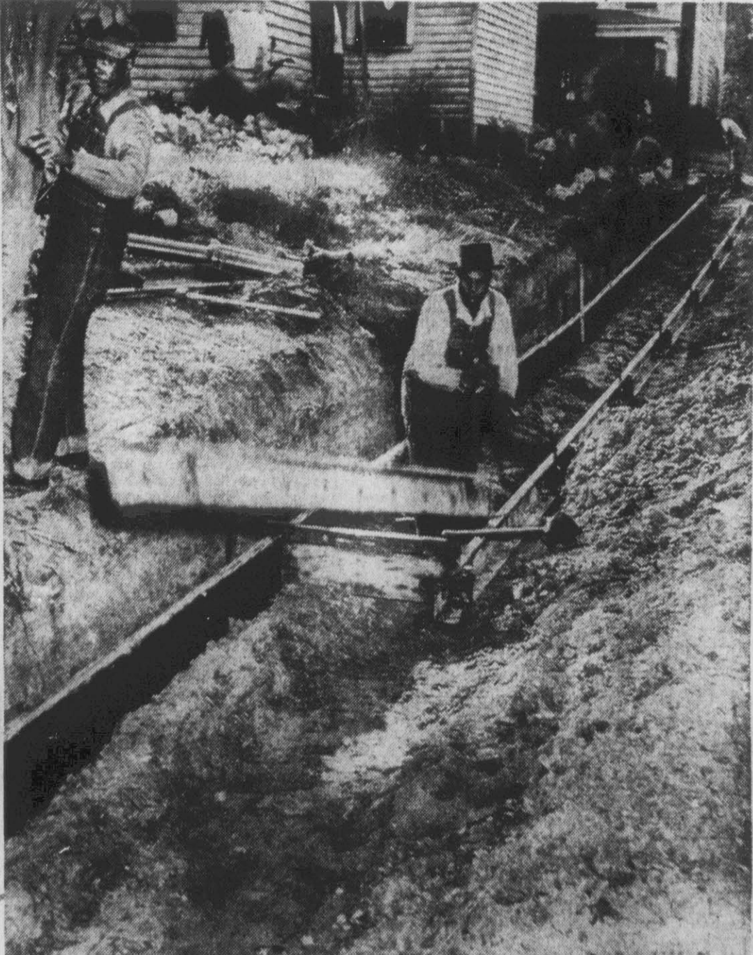
Before a street can be paved, work crews lay the curbs and install the necessary drainage facilities.
