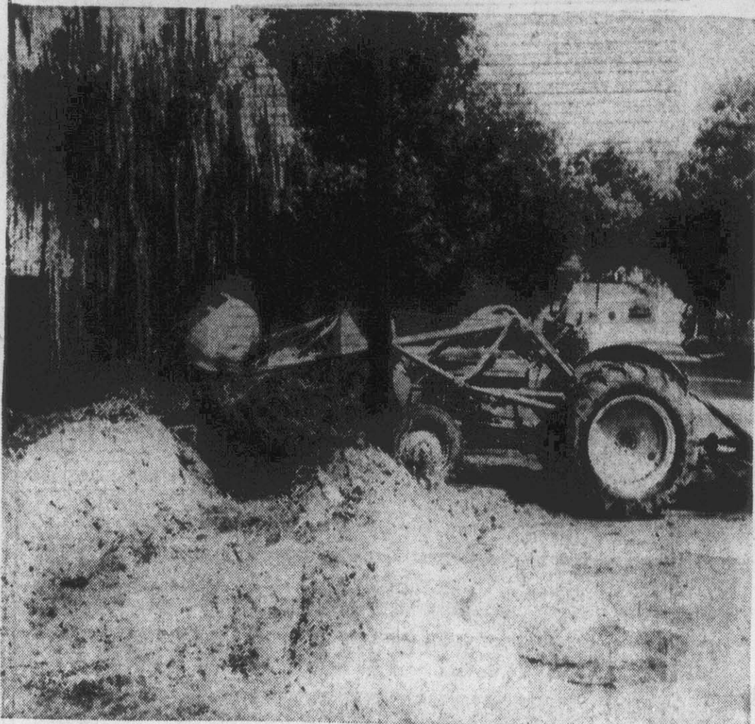
Sidewalks will soon be on the sides of Third Street, between Summit and Cotanche, as the street department is rapidly constructing the new sidewalks. Above a department machine levels the ground in preparation for completion of the job. (Reflector Photo by Roy Hardee).
