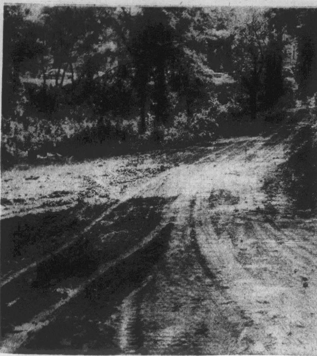
A new parking lot to aid the congested traffic situation in Greenville is rapidly taking shape in the ravine between Fourth and Third Streets near the high school. Already a road has been cut connecting the two streets, and work is in progress on the parking lot itself. (Reflector Photo by Roy Hardee).
