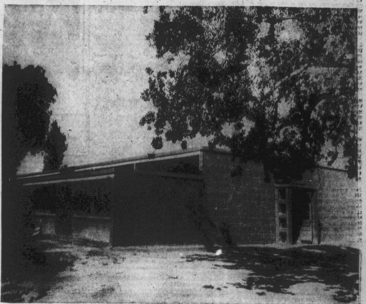
Including equipment, this new eight room building at the Pitt County Training School cost around $70,500. The building is heated with steam, equipped with new desks and chairs, and has modern toilets. (Reflector Photos by Roy Hardee).
