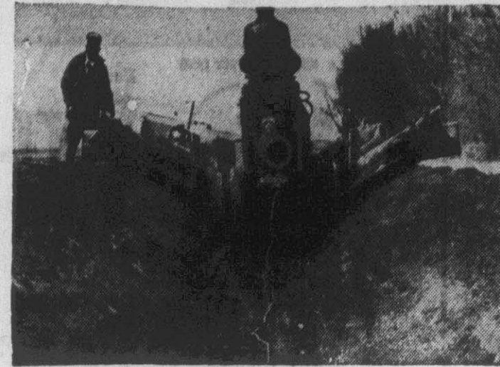
A PLOW-TYPE ditch-digger prepares the canal for lining.
