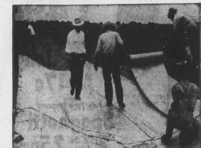
STRIPS of fiber glass are laid like carpets and an asphalt membrane is created by spraying with a hot solution.
