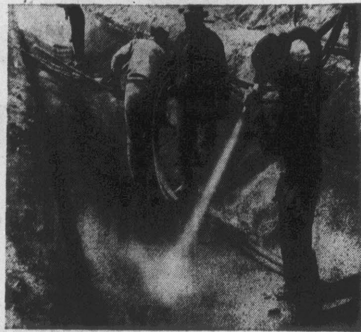
SHOTCRETE, a concrete mixture blown on with air pressure provides a smooth floor in the canals.
