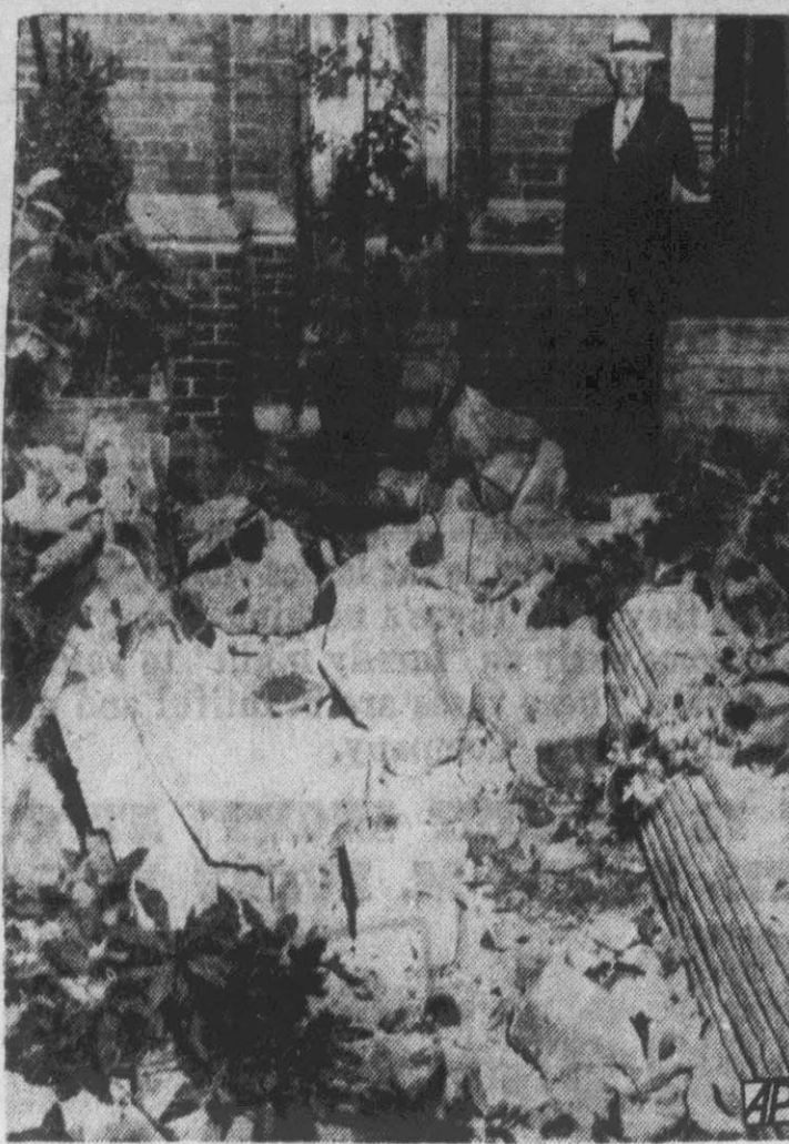
A. T. Brown, building superintendent, inspects damage in patio of the Glendale, Calif., Presbyterian Church. Debris in foreground is from one of the church spires which fell during early morning earthquake. Several persons are known to be dead from the quake which shook a large section of California. (AP Wirephoto)
