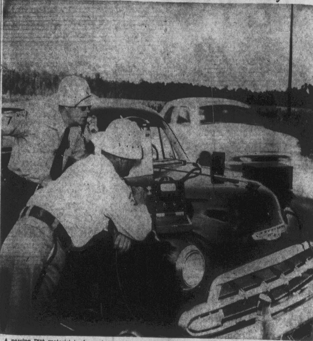
A passing Pitt motorist is shown being clocked by the radar control speed meter which was operated in this area yesterday by the Highway Patrol. In the above picture, Lt. Tom Brown (center) checks the speed of the passing car while Patrolman Dillard, of Kinston, radios ahead for the car to be stopped for traffic violation. The black box, located on the left fender of the car, is projecting the radio waves which "bounce back" the speed of the cars. (Reflector Photo by Roy Hardee)
