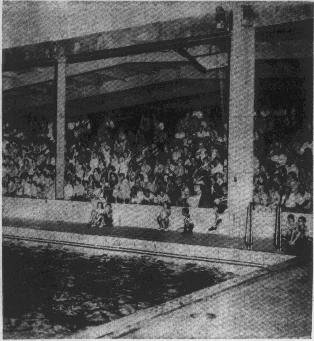
The new health and physical education building was opened last night when a reception was held. Here a portion of the attending crowd is sitting in the bleachers of the main part of the building. The modern swimming pool is shown in the foreground. (Carolina News Bureau Photo).
