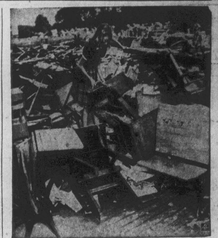
SCHOOL'S OUT EARLY: —Eleven-year-old Barbara Ann Stinson, a sixth grade student, hunts for her books in the rubble of the grammar school after a tornado whipped through the south Georgia town of Alapha. Vicious winds leveled sections of the town of 600 persons and caused heavy property damage. No one was killed; three persons were hospitalized. Mayor Julian J. Paulk estimated property damage would approach a half-million dollars. (AP Wirephoto).
