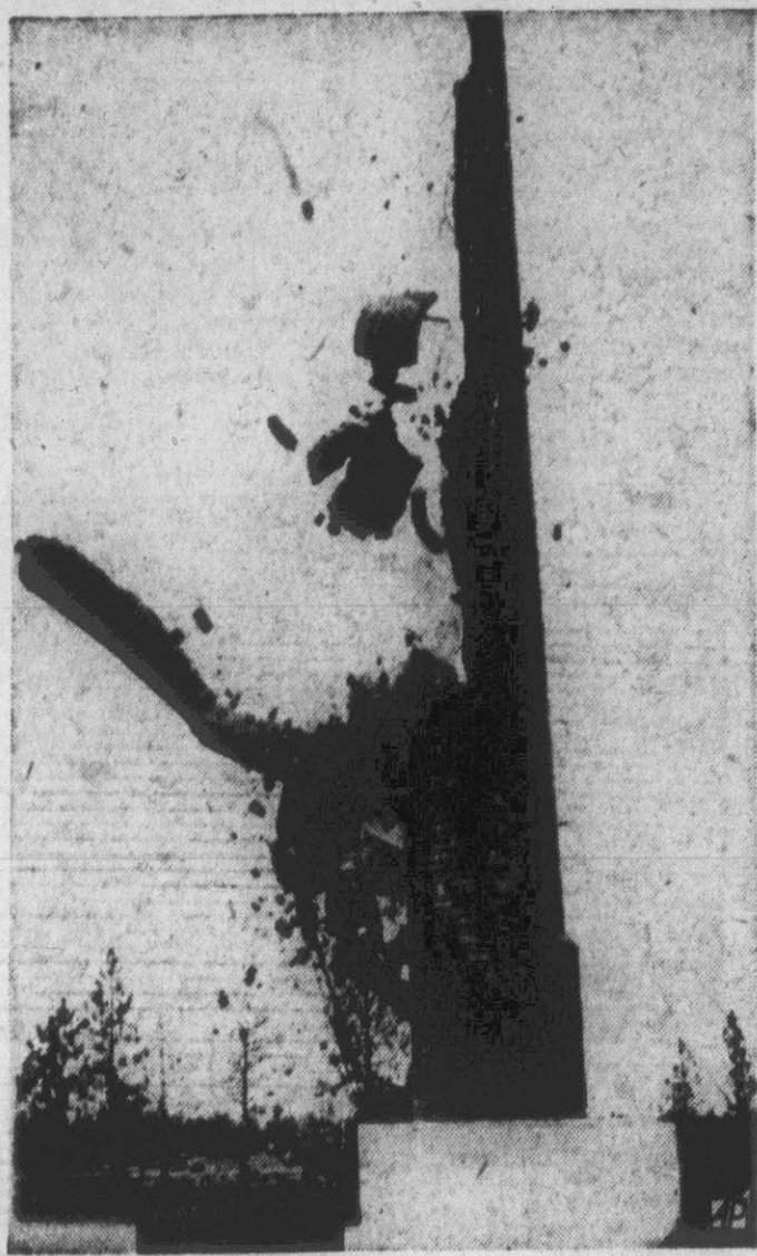
FINALLY FALLS:—A winch-powered block and tackle finally pulls down sturdy, unused 100-foot chimney at Spokane, Wash., that was damaged by a lightning bolt. Firemen blasted remains twice with ten sticks of dynamite, pulled it with thick cable, fired at it with strong water pressure. Stack remained standing until the block and tackle were used. (AP Wirephoto).
