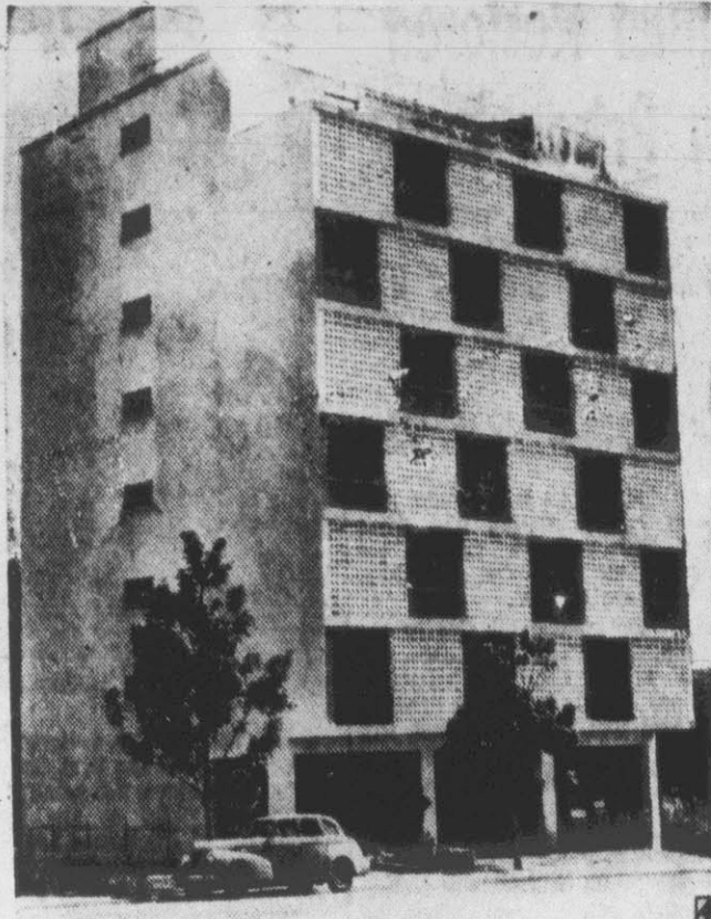
MODERN DESIGN —Beehive brick design on the balconies of apartment house development in Caracas, Venezuela, creates a natural air flow and protection from the tropical sun.
