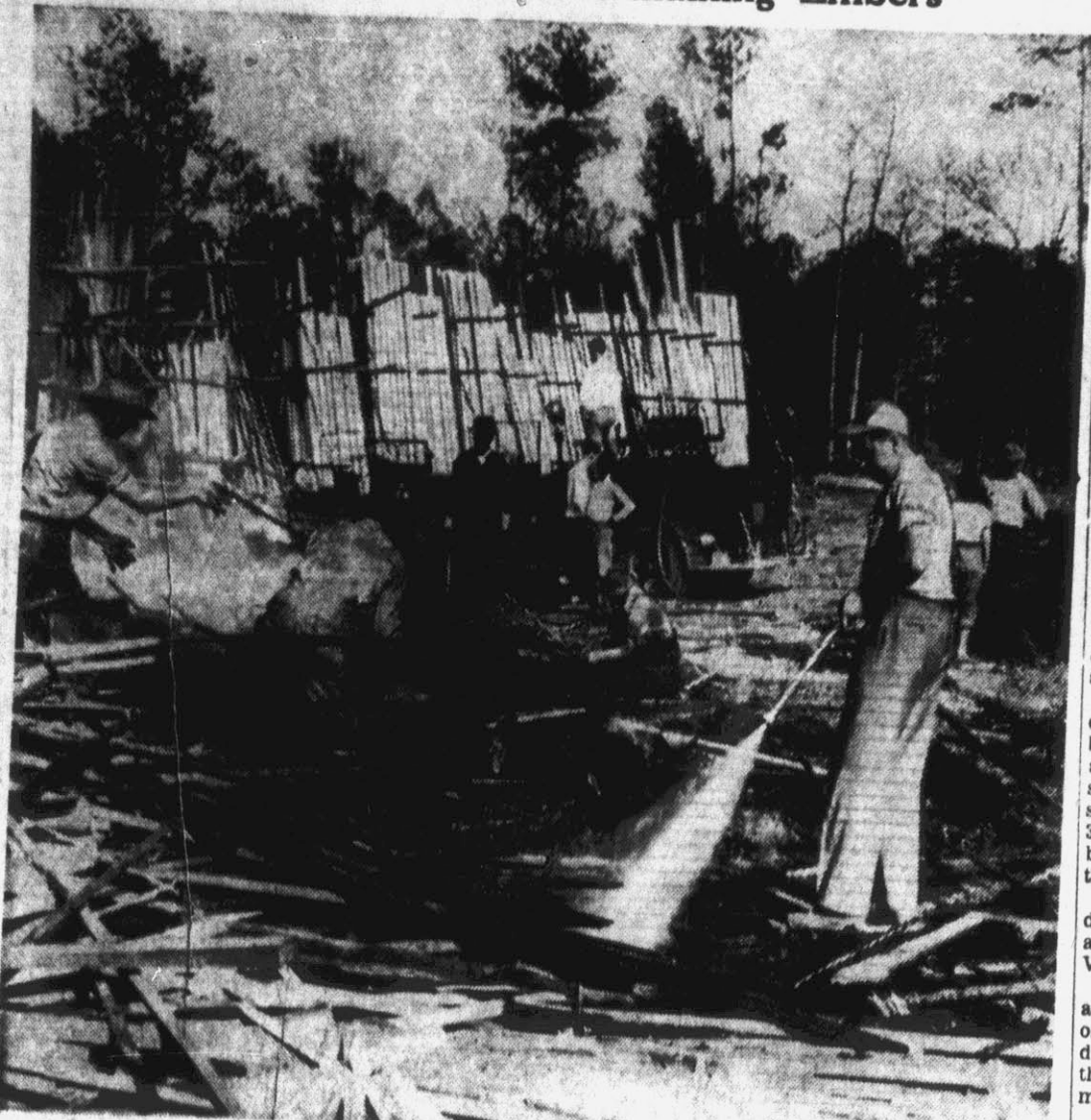
Fire fighters are shown as they tear through burned timbers in an effort to put out any remaining flames at the R. G. and W. E. Little Lumber Company Saturday afternoon. Prompt work on the part of volunteer workers and Greenville firemen prevented the fire from reaching the main buildings of the mill. (Reflector Photo by Roy Hardee).
