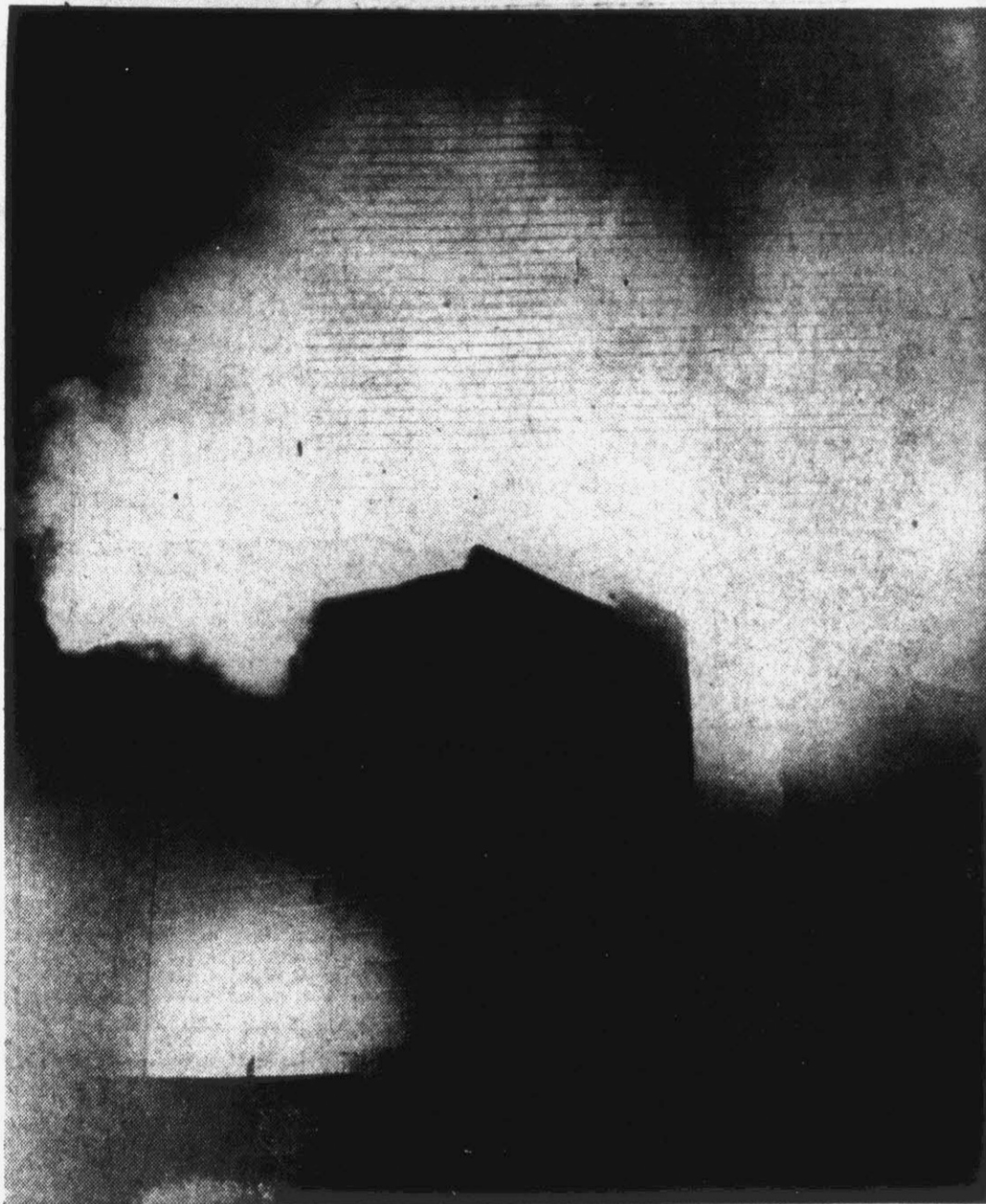
Flames and smoke bill high into the air as an early morning fire gutted Overton's Super Market on the corner of Third and Jarvis Streets. The blaze, discovered just before 4 a. m., had broken through the roof of the structure before being noticed. Neighbors were awakened by popping sounds coming from the burning building. (Reflector photo by Roy Hardee).
