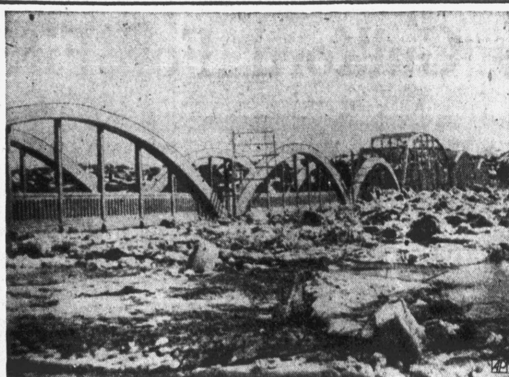
ICE JAM SMASHES NEW BRIDGE:—A huge, 82-mile long ice jam in the South Saskatchewan river piles against this 1,215-foot bridge at Swift Current, Sask., in Canada, shortly before the pressure became too great and three spans were torn from the center and disappeared into the churning river. The $1,000,000 bridge was built last year. (AP Wirephoto).
