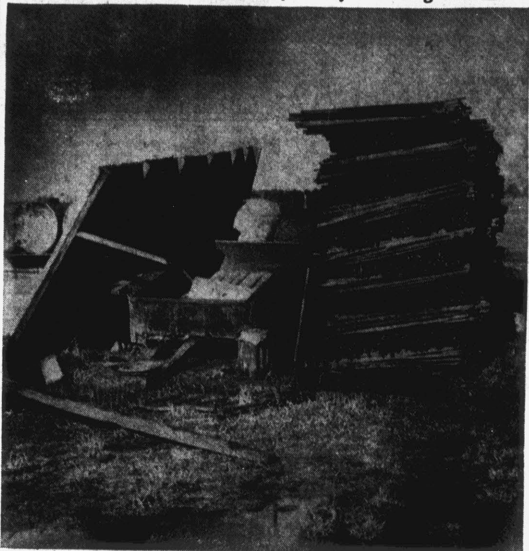
The contents of this destroyed shelter barn on Mrs. Celia Harris' farm near Ayden was left undamaged early this morning by a gale-like storm which roared out from the West and ripped the building down. The top and side of the building were blown across the Ayden-Grifton highway blocking traffic there for some time. Other reports of tobacco barn tops being blown off were heard in the county. (Reflector Staff Photo by Roy Hardee).
