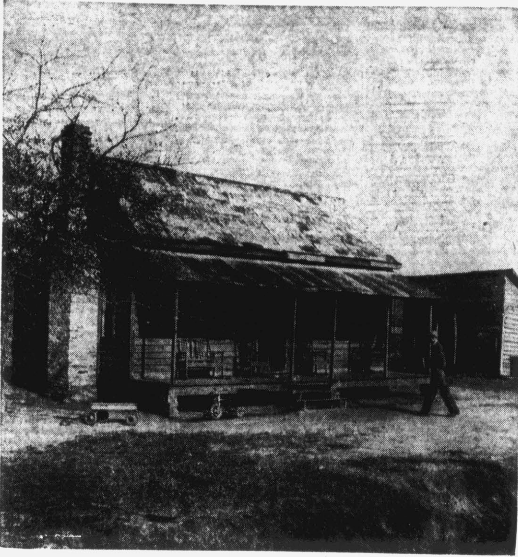
This three-room cottage in which the Fleming family has lived since 1914 will be vacated by them around the first of April. They have rented this house for the past eight years, but within a few weeks they will move into a new and roomier structure, built for and dedicated to them by their neighbors at Stokes.
