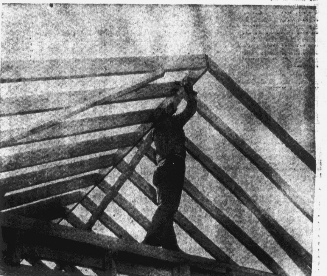
A workman puts the finishing touches on the "ridge pole" in the house the community is building for John Fleming. The six-room structure will be weather boarded with cypress "german siding," and the entire inside will be finished with paneling of knotty pine. It will be completed around the first of April.
