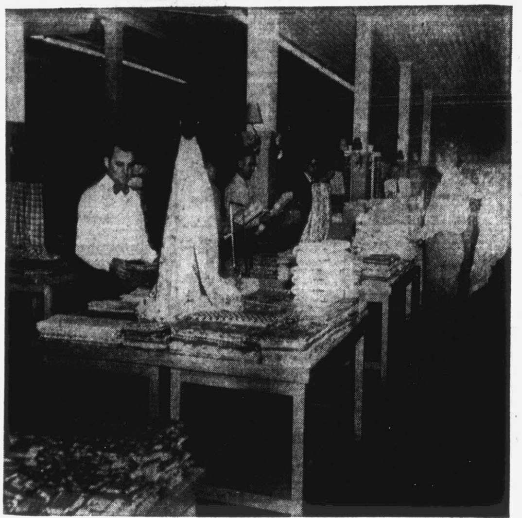
Greenville's newest department store will open its doors for business tomorrow morning at nine o'clock. In the picture shown above, clerks and stockers are shown placing merchandise on counters in the firm's new store. The new store is located at the intersection of Dickinson Avenue and Green Street. (Reflector Staff Photo by Roy Hardee).
