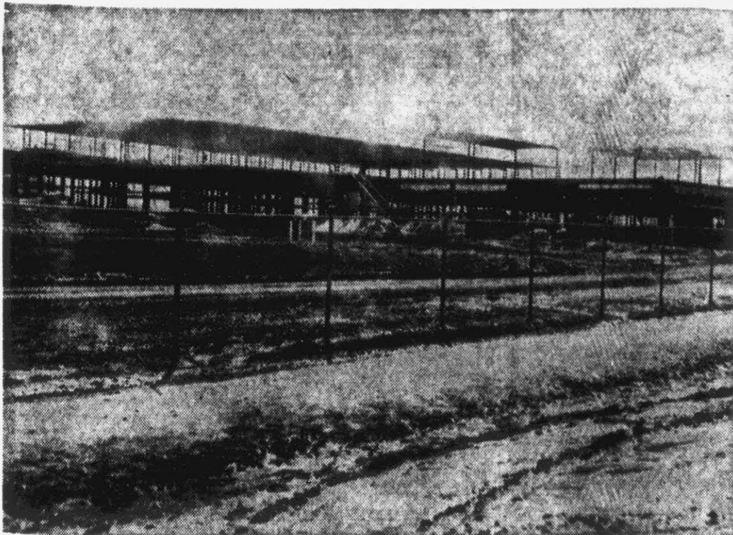
Construction workers of the multi-million Du Pont Plant near Grifton began returning to their jobs this morning following the announcement that the dispute between the company and the painters' union had been settled. The photo above was taken during the five-day picketing of the plant site which threw some 900 construction workers out of their jobs. The plant site took on new life this morning as the workers returned to their tasks of constructing the buildings which are being erected near Grifton. (Reflector Staff Photo)
