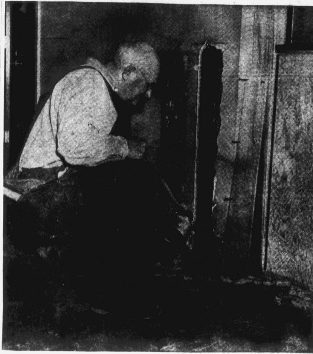
OLD MAN TERMITE IS LOSING his battle of destruction he has waged at City Hall for many months. Above, a workman is shown giving the insects (if any remain) a poison spray before completing repairs to the interior of the building which had been heavily damaged by the voracious insects over a period of years. —(Reflector Staff Photo by Roy Hardee)
