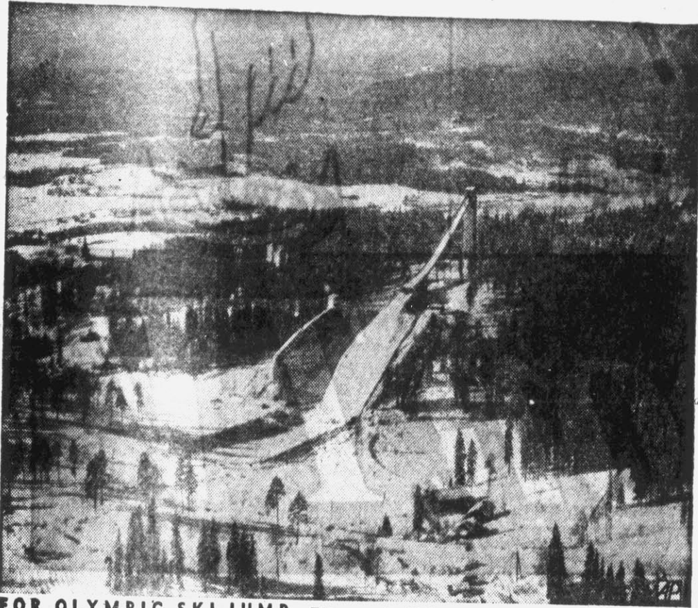
FOR OLYMPIC SKI JUMP —This concrete, 33-degree, 168-foot runway on Holmenkollen Hill near Oslo, Norway, will be the scene of the 1952 Winter Olympics ski jumping tests.
