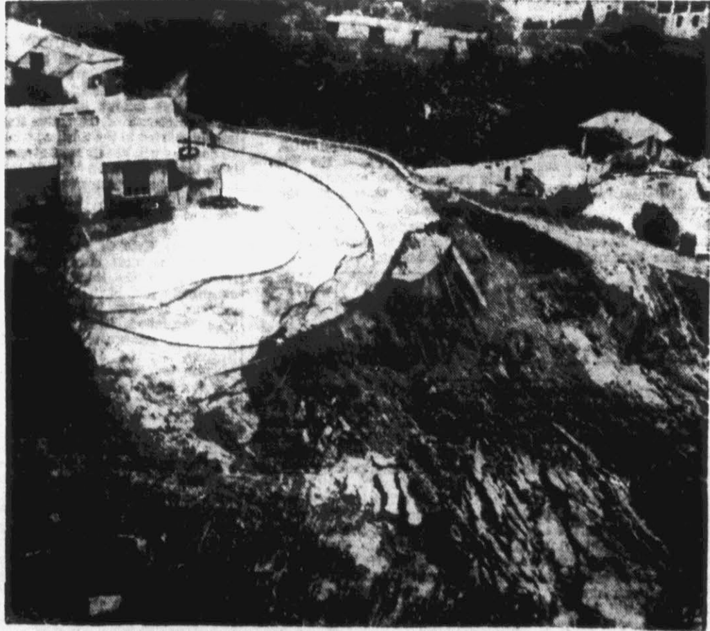
MUD SLIDE PERILS HILLSIDE HOMES:—A deluge in waterlogged southern California caused this landslide next to the home (upper left) of Paul Franklin in Pacific Palisades in Los Angeles, Calif., and threatened destruction of his swimming pool. The soggy earth slide across the coast highway and blocked it to traffic. All highways in and out of Los Angeles County were reported impassable after three days of torrential rains. (AP Wirephoto)
