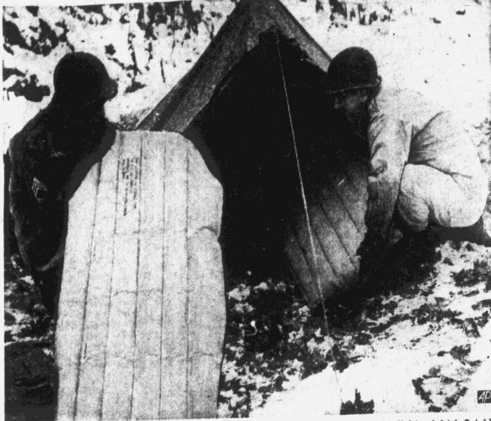
SUPER SACKS —U. S. servicemen in Far East are to be equipped with lightweight inflatable sleeping pads of nylon fabric and rubber, treated to resist cracking in cold weather.
