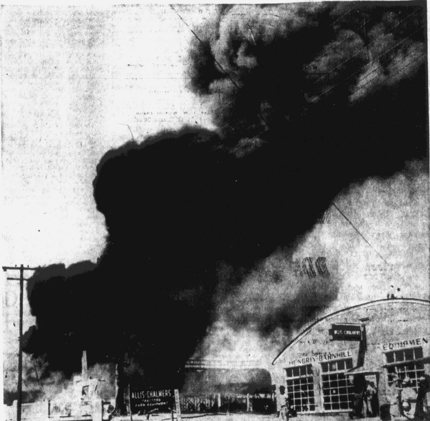
Fires took a high toll last year, when over $400,000 went up in smoke in the city of Greenville. Shown above is a spot picture of the Sinclair Oil Company blaze. The fire was one of the most threatening fires to hit the city in some time, as several other oil companies were located nearby, but were kept from damage.
