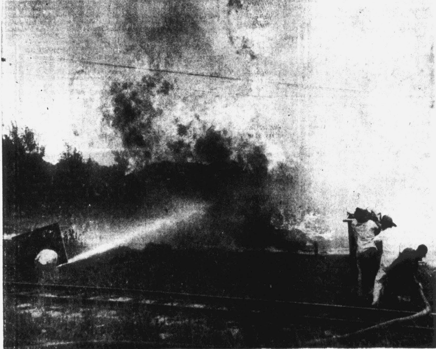
Damage estimated at over $125,000 was caused when the Perkins Lumber Company, of Greenville, was razed by a summer blaze which taxed the city's fire fighting ability to the limit. In the above photo, firemen pour water on the blazing lumber yard from behind barricades, in order to protect themselves from the heat.
