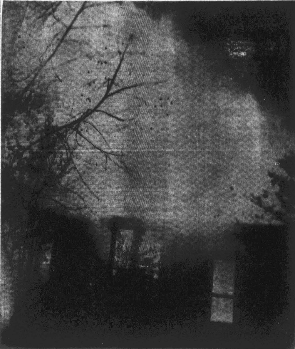
Wind-ted flames soared upward from a blazing seven-room home destroyed by fire early Sunday morning. Six persons, including three small children, escaped the fire clad only in night clothing. Nothing in the house was saved. A second home nearby was heavily damaged. (Reflector Staff Photo by Roy Hardee).
