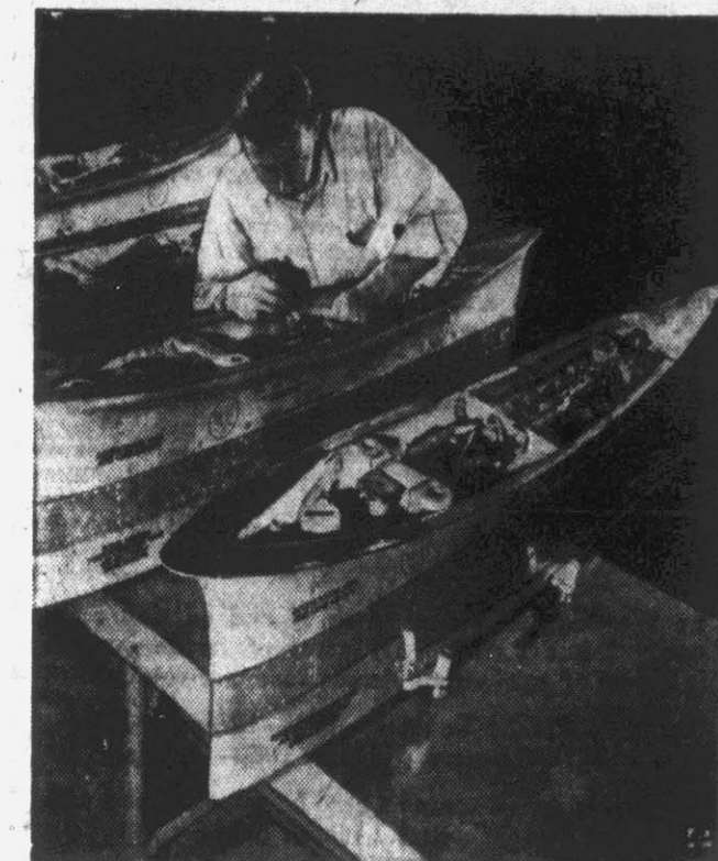
WING WINDUP—John Heuss checks a pylon at Mansfield, O., factory before shipment to jet plane assembly plant for suspension beneath wing as part of fuel or armament system.
