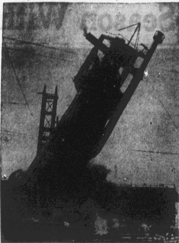
CASUALTY OF PROGRESS—Dynamic and a steel cable attached to a locomotive send this blast furnace toppling during renovation of the Minnesota Works in Pueblo, Colo.
