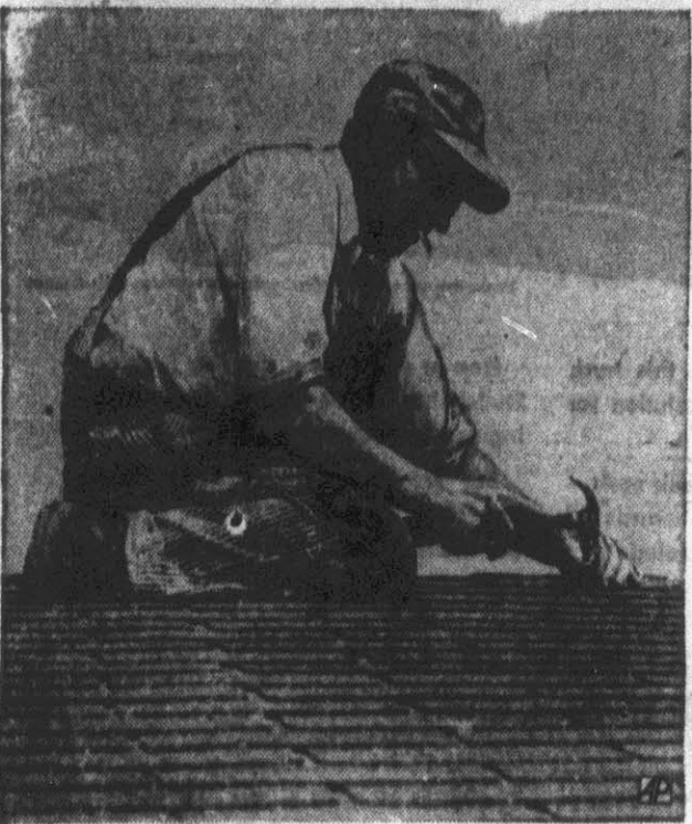
CARPENTER WITHOUT SIGHT—Alex Meuwissen, blind carpenter of Chaska, Minn., lays ridge shingles on house roof depending upon developed senses of touch and hearing.
