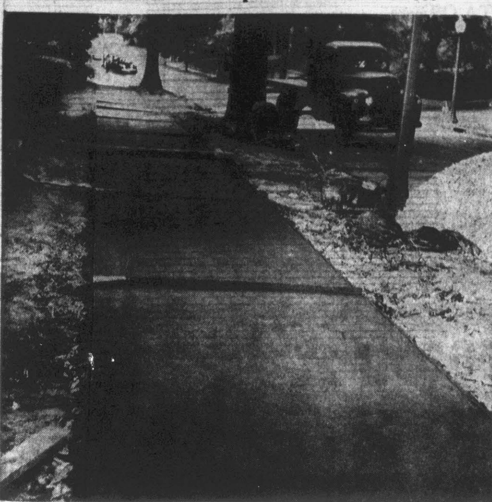
No longer do college students and townspeople alike have to stumble along the broken sidewalks which once lined Fifth Street in front of East Carolina College. Now the city has removed the old sidewalks, moved them back and poured new cement walk-ways which were completed yesterday. Work was done by the City Street Department. (Reflector Staff Photo by Roy Hardee).
