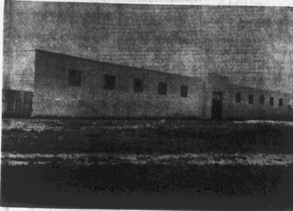
Pictured above is the new exhibit building at the new Pitt County Fair grounds on the north side of Tar river near the airport. Workmen are busy putting the finishing touches to the interior of the building in preparation for the opening of the annual Pitt County Fair sponsored by the American Legion. The fair this year will be the week of October 1. The dedication of the new fair grounds will be held Tuesday night. (Reflector Staff Photo.)
