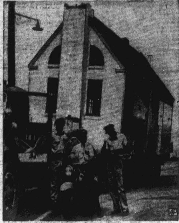
'TAKE IT AWAY, PLEASE'—Birmingham, Ala., highway police discuss dismantling of this house during removal to another site. When told it would block highway, police consented.
