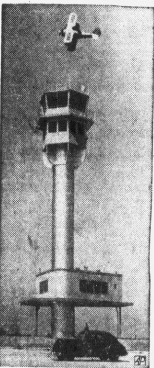
AERIAL PERCH — Control operators will get a bird's eye view of traffic from this new 100-foot-high tower being completed at Sky Harbor Airport, Phoenix, Ariz.
