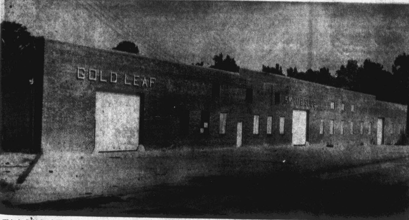
This is Gold Leaf Warehouse which was sold Thursday for the highest amount ever paid for such a building in the world. Located at the intersection of Charles and 14th Streets, it comprises 76,000 square feet of floor space, making it the sixth largest warehouse in Greenville. By this morning no one had raised N. G. Raynor's bid for $198,000. (Staff Photo By Roy Hardee).
