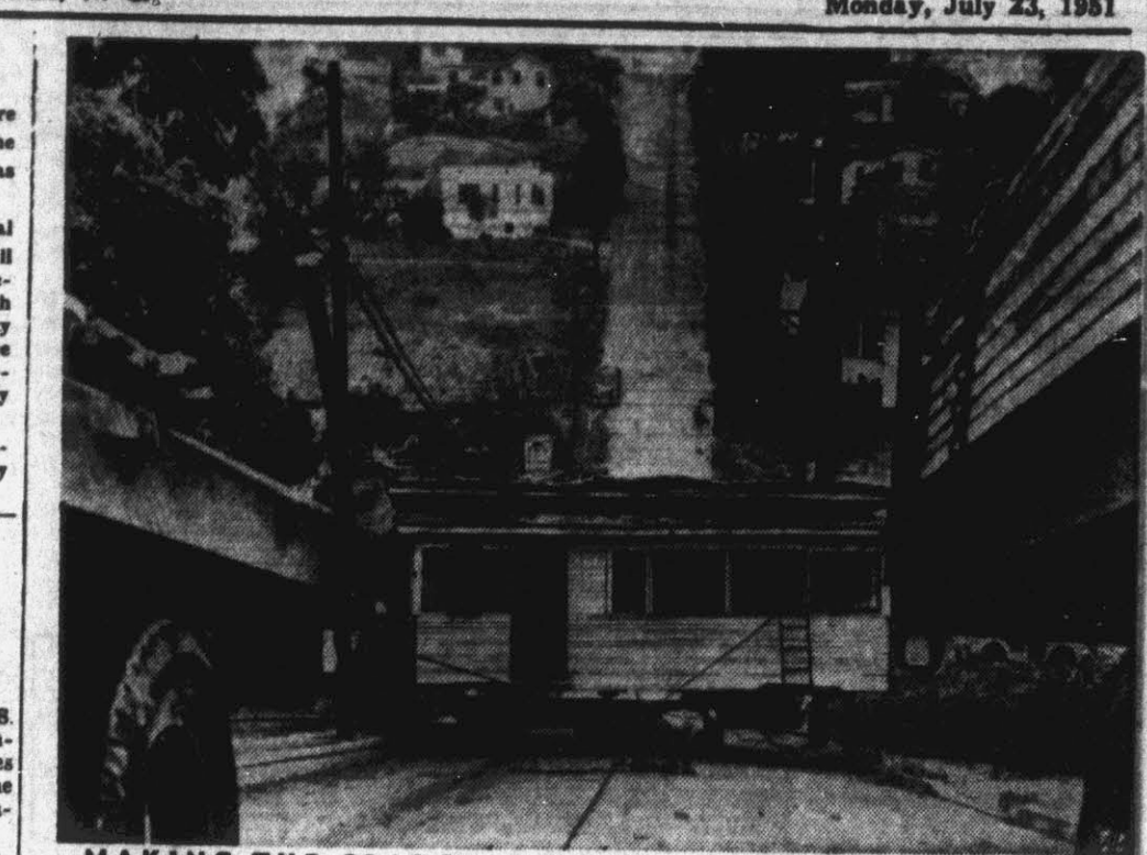
MAKING THE GRADE—A six-room house is inched up one of Los Angeles' steepest grades with use of winches by two trucks, each anchored to manholes and telephone poles.
