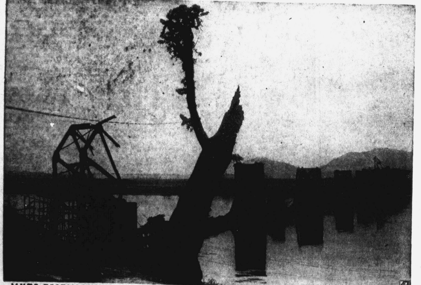
MUTE TESTIMONY TO FURY OF WAR—A shattered tree stands like a gaunt sentinel before the war-wrecked remains of a bridge over the Han River, a natural barrier on the western front in South Korea.
