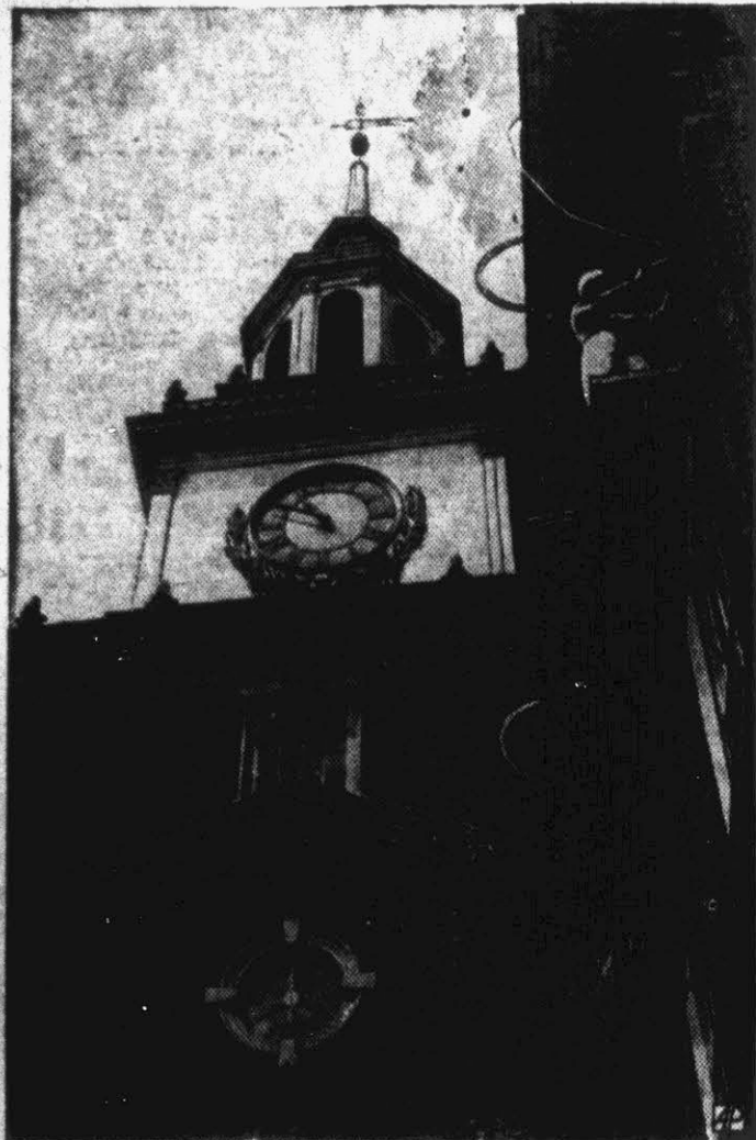
REMOVING RAVAGES OF TIME — A worker points bricks of historic Independence Hall, Philadelphia, as face-lifting operation on the American shrine gets under way.
