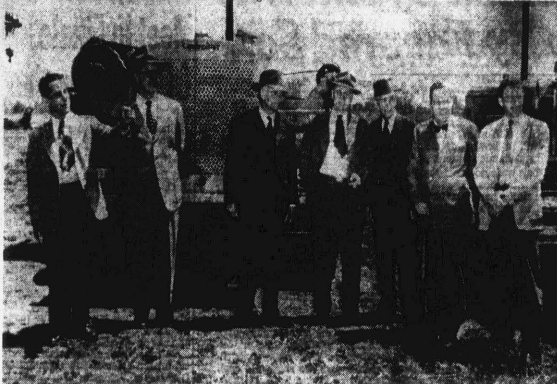
C. S. Anderson (left) Du Pont field project manager who is in charge of the construction of the new $33,000,000 Dacron plant near Grifton, points out things of interest on the building site to a group of Pitt countians who yesterday attended the ground-breaking which marked officially the beginning of the construction on the project.
