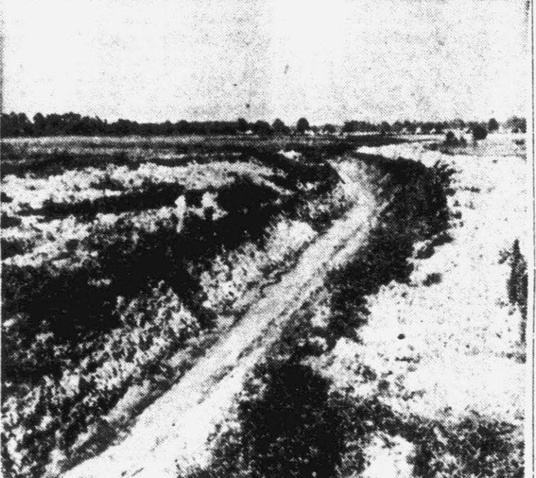
Canals such as the one shown above are needed often times to drain the excess water coming from tiled fields. Correct planning and construction of the canals is carried on by the Soil Conservation department, with labor furnished by the farmer.
