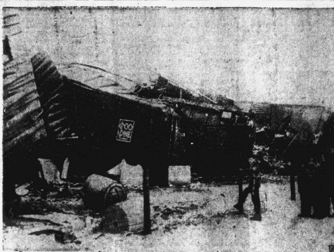
NEWSPRINT GROUND TO PULP—A section of 43 freight cars are piled up in a fantastic jumble on the Soo line near Duplainville, Wis., Saturday. Most of them were loaded with newsprint. The mishap occurred at a siding when as one freight train waited for another to pass. Forty-three cars of one train were derailed as well as the locomotive of the other. No one was injured. (AP Wirephoto).
