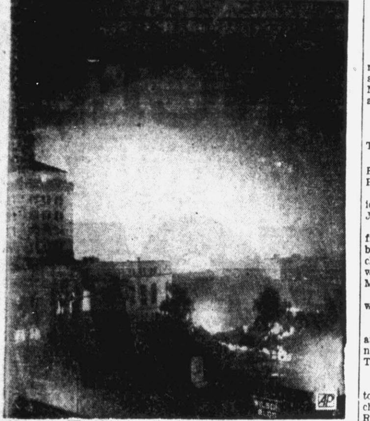
ATOM BLAST.—Light from Tuesday's atomic explosion in the Nevada desert nearly 300 miles away pierces the fog and outlines the City Hall tower (left) in Los Angeles, Calif. This picture is a time exposure made from the top of the Los Angeles Times building by Photographer John Malmhin of the Times. Pre-dawn darkness gripped Los Angeles at the time of the brilliant flash in the eastern sky. (AP Wirephoto).
